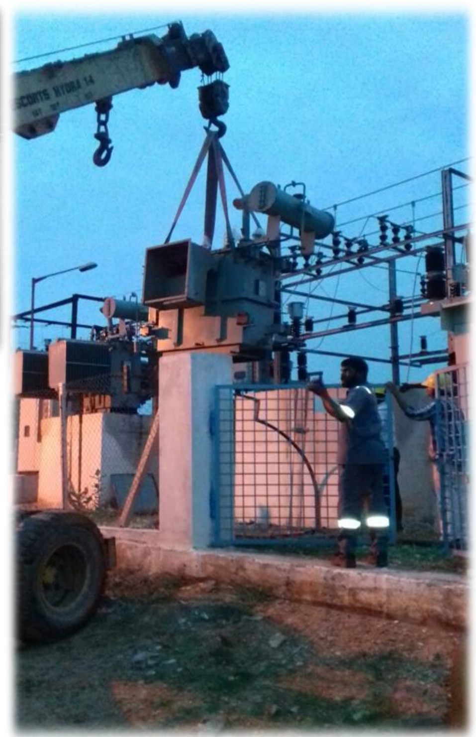
Provided Machinery and manpower for the electrical installations of Lift Pump
