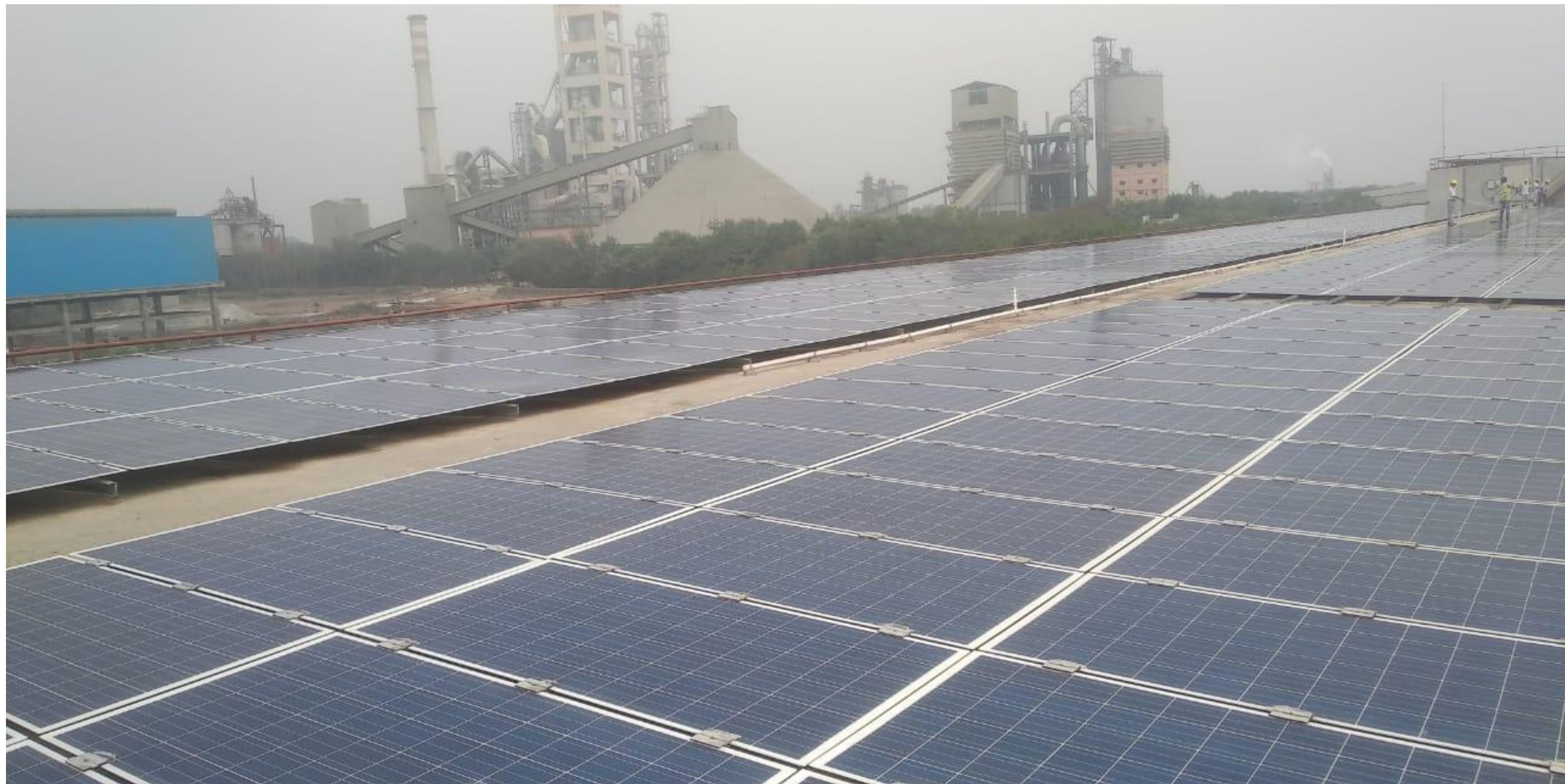
Photo of Solar Panels arrangement on Roof Top of Railway Wagon Shed. (1.2 MW)
