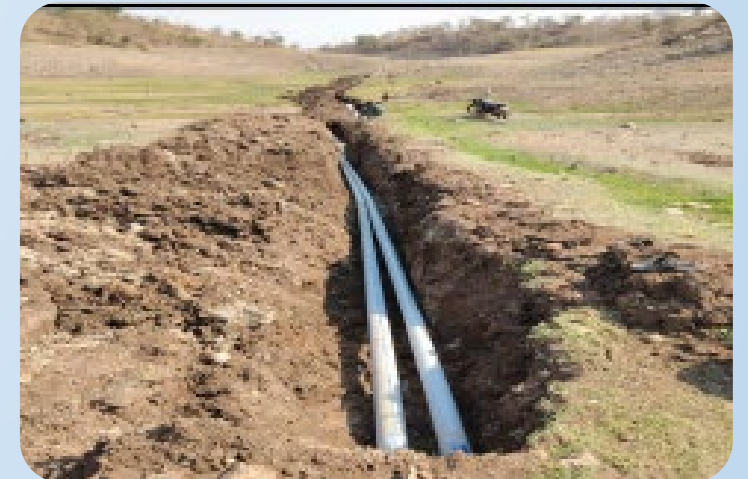
Laying of 72 PVC pipes for increasing water availability to support agriculture in Rodada panchayat, near Jeerabad
