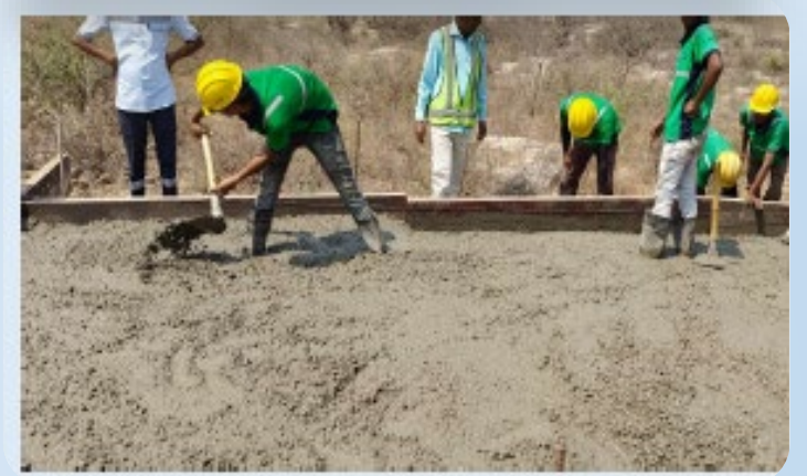
Laying of CC Road At Ramapuram Village at Dachepalli
