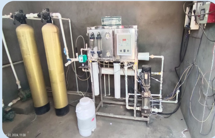
Installed RO based-Drinking Water Cooler in Durga Public School, Dachepalli, Andhra Pradesh.
