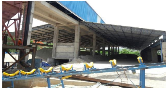
Raw Material storage facilities
