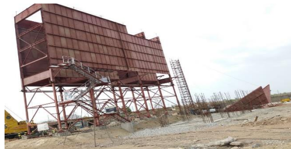
CPP - Electro static Precipitator & BOILER
