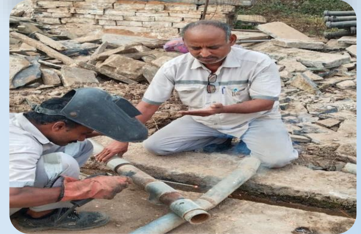
Drinking water pipeline repairing work undertaken under CSR
