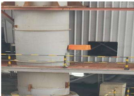
Opacity Meter(Coal Mill Stack)
