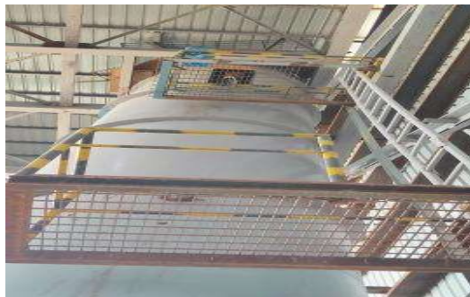
Opacity Meter (Cement Mill Stack)
