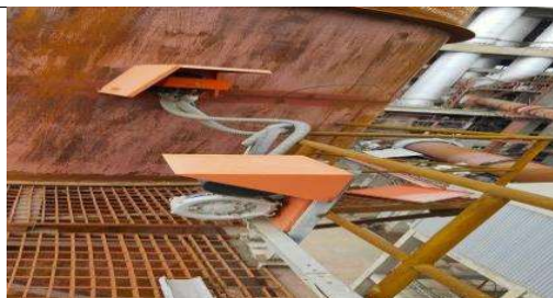
Opacity Meter(Cooler ESP Stack)
