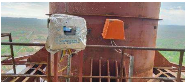
Opacity Meter (RM+Kiln Bag house Stack)
