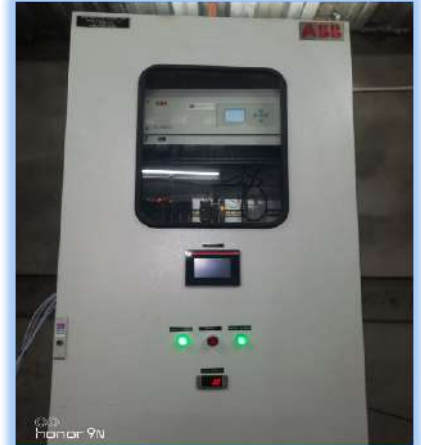
CEMS (Continuous Emission Monitoring System) with Analyzers
