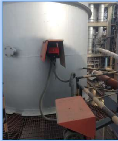
CEMS (Continuous Emission Monitoring System) with Analyzers
