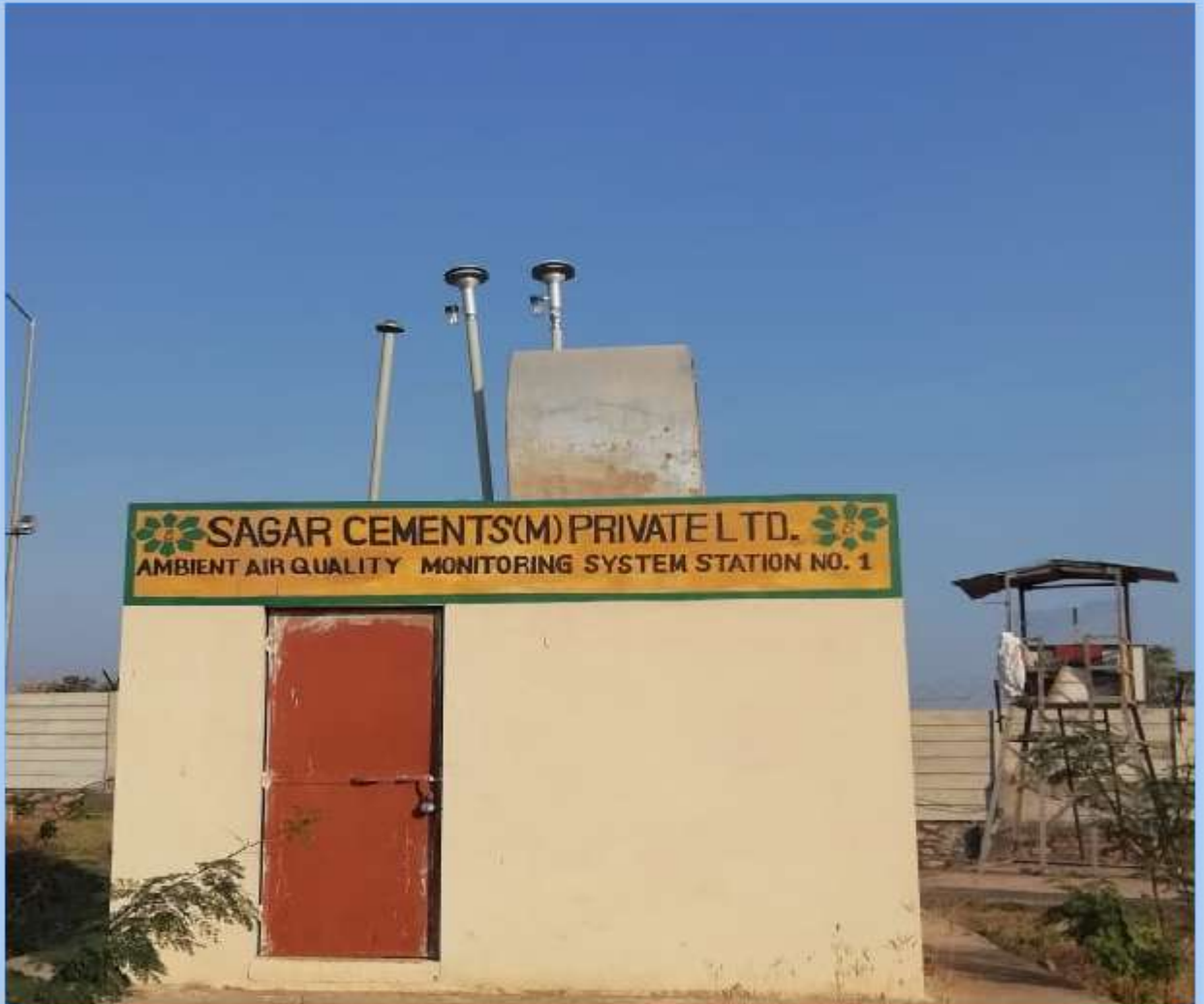
Continuous Ambient Air Quality Monitoring System (CAAQMS) installed and Connected to the Central Pollution Control Board & MPPCB.
