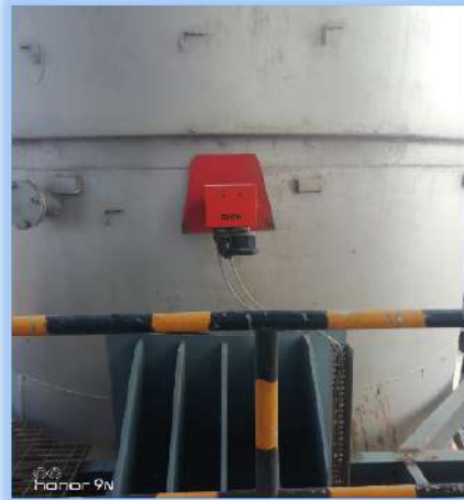
CEMS (Continuous Emission Monitoring System) with Analyzers
