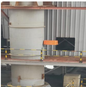
Opacity Meter(Coal Mill Stack)
