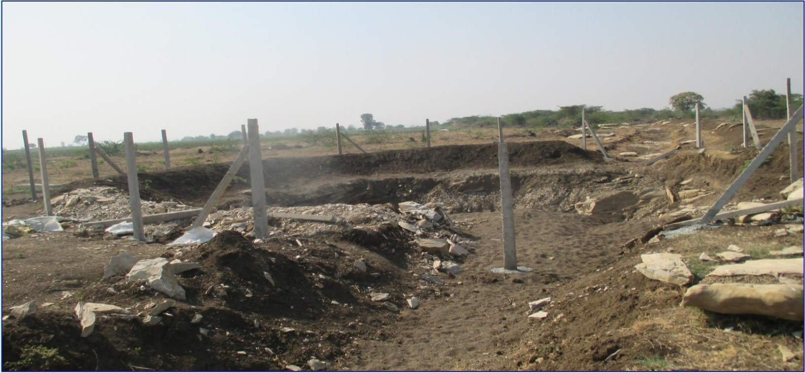
Silt Settling Tanks constructed across the Garland Drain
