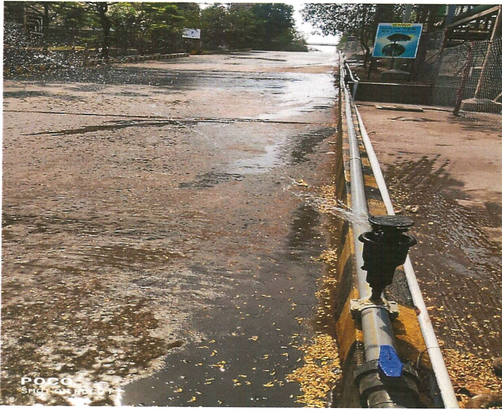
Image: Showing water sprinkler systems at road side
