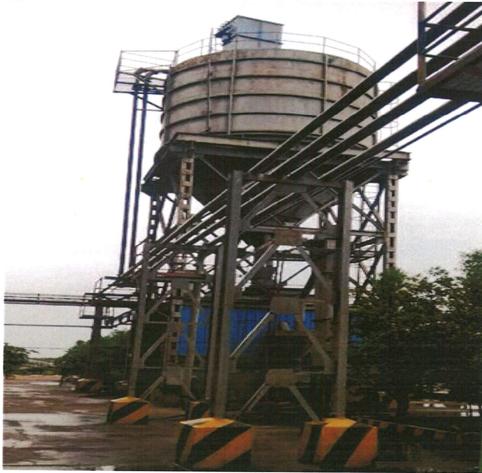
Image: Showing Bed Ash Silo
