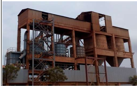
Raw material silo
