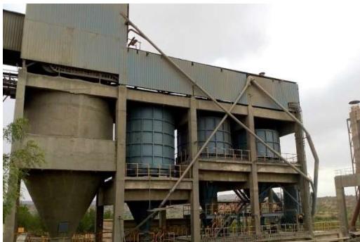
Raw material Silo
