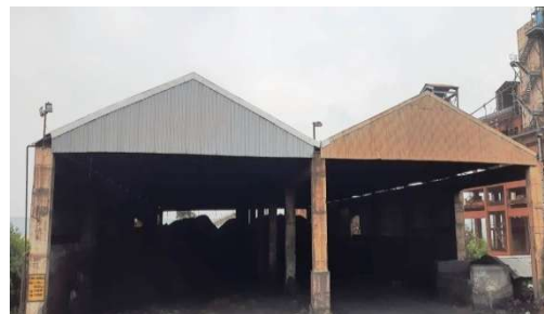
Coal Sheds at Cement Plant
