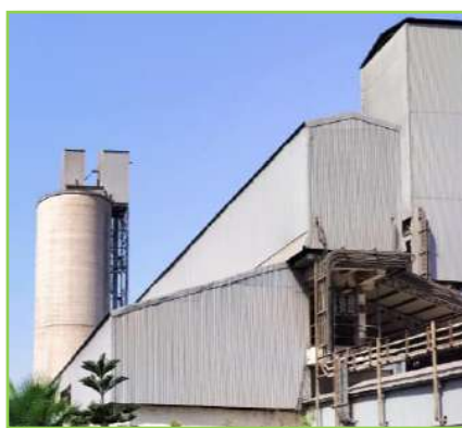
Concrete silo for Clinker storage
