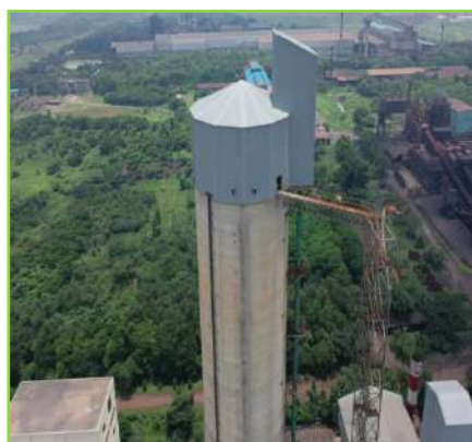
Concrete silo for product storage
