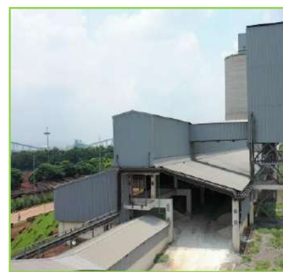
Raw Material storage shed
