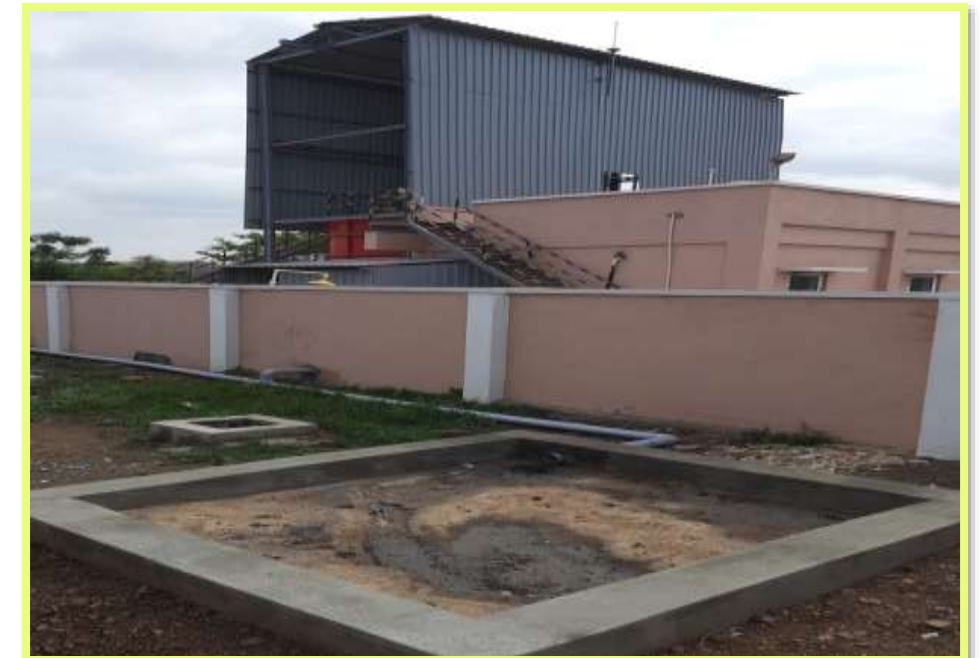
Rain water harvesting pit near Plant area
