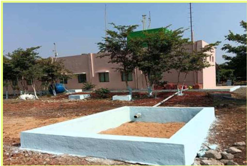
Rain water harvesting pit near Mines Office
