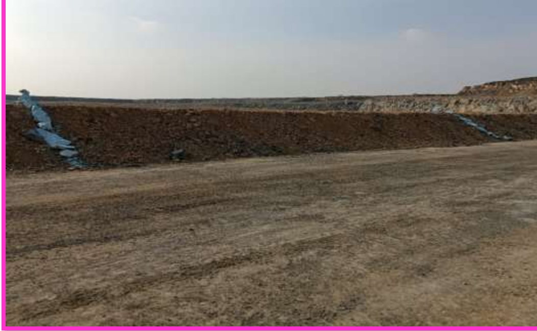
Bench Floor and Burm maintained East side
