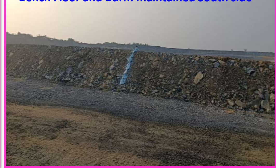
Bench Floor and Burm maintained South side
