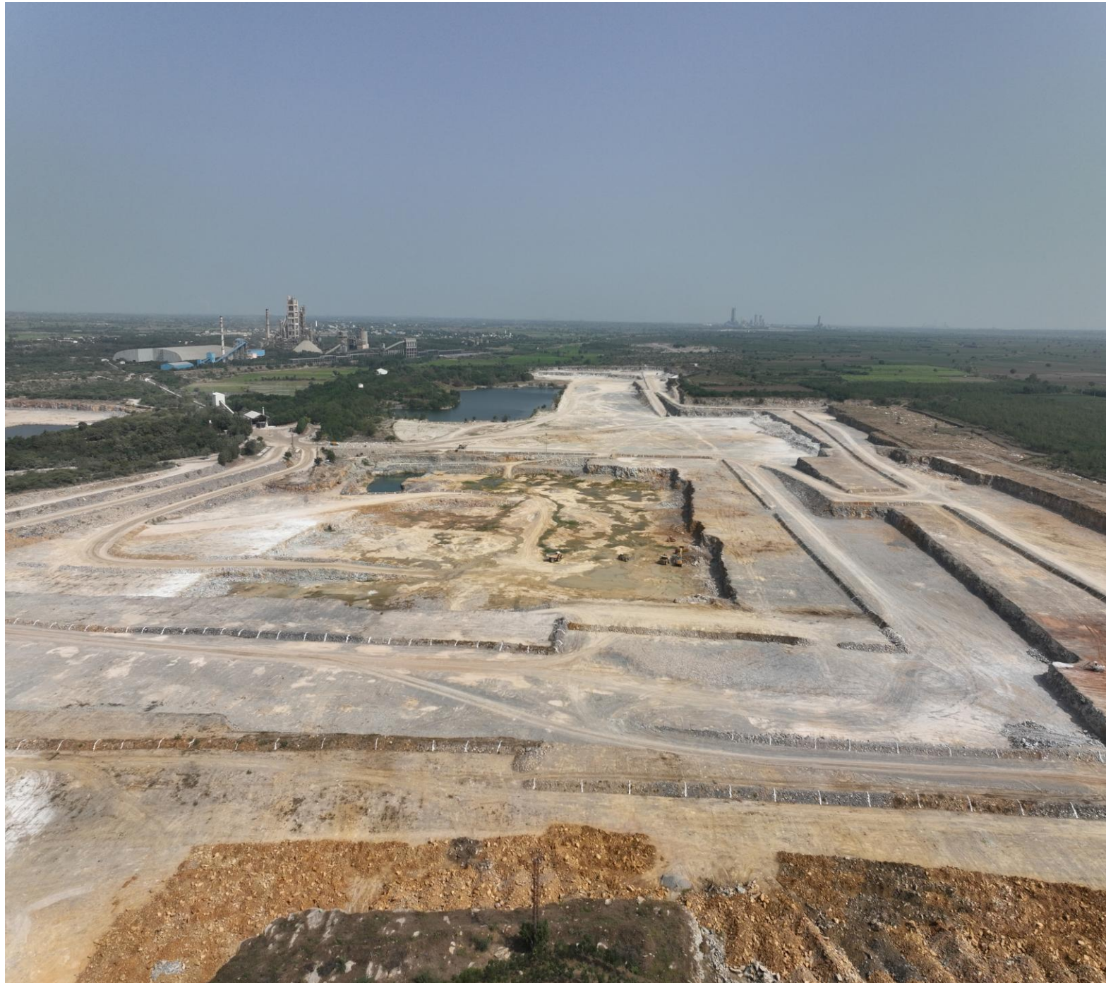
Sagar Cements Limestone Mine-I
