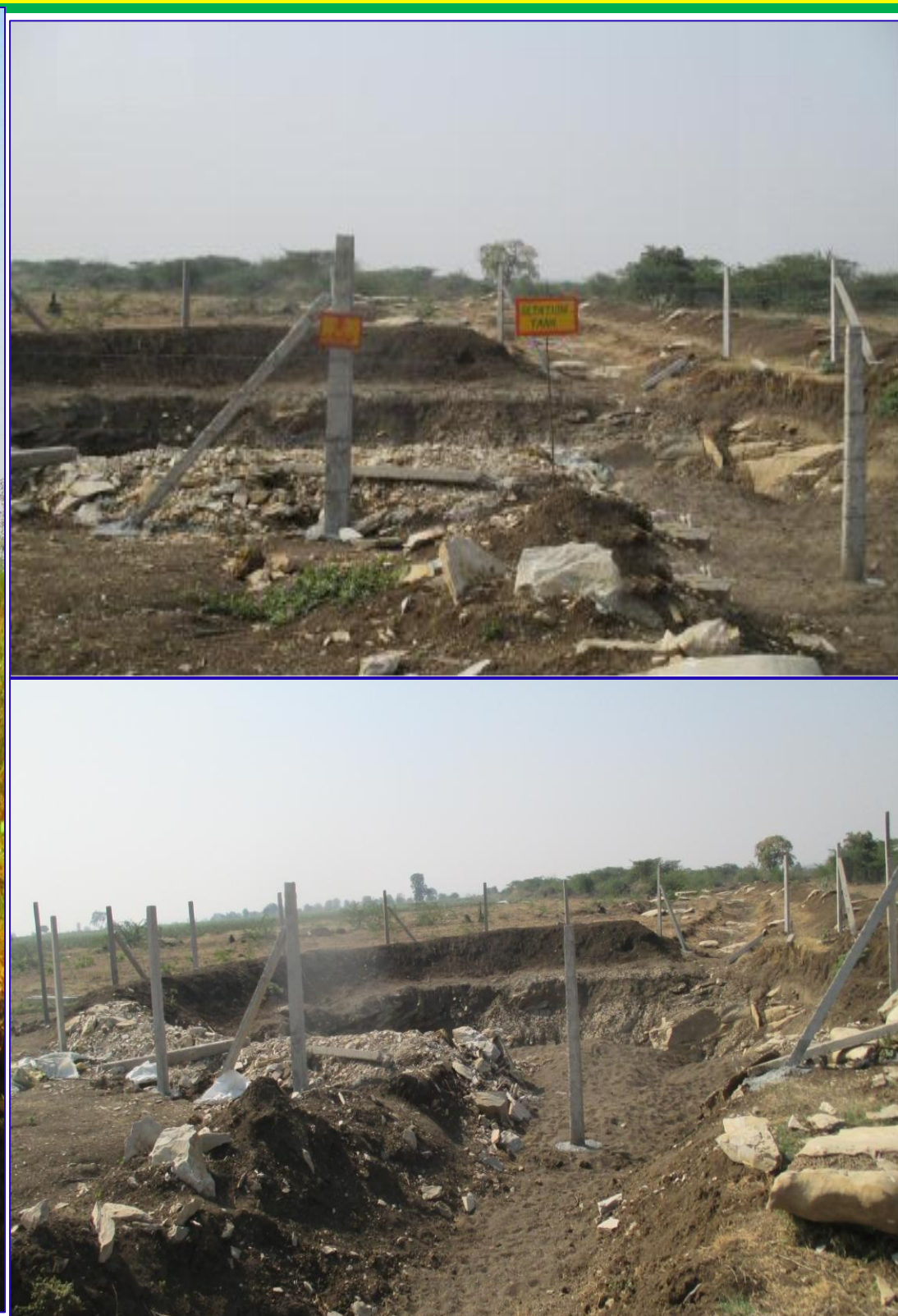
Silt Settling Tanks constructed across the Garland Drain
