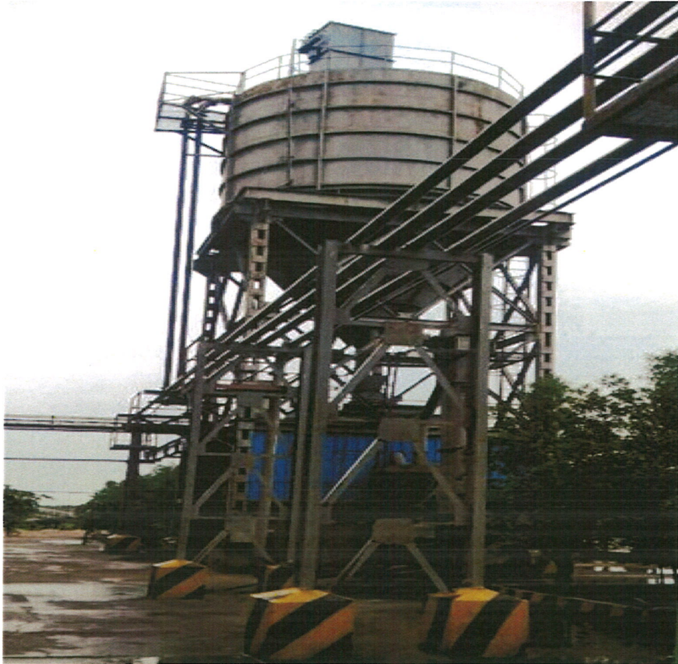
Image: Showing Bed Ash Silo
