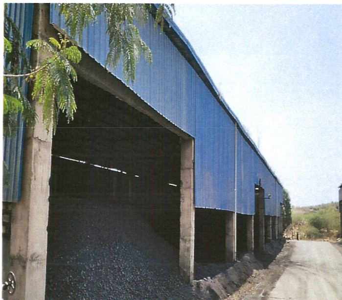
Image: Showing 2 no's of Coal Sheds of capacity 5000T each
