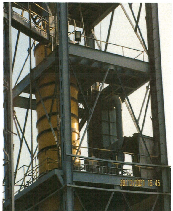
Image: Showing Dust extraction system to control fugitive emissions
