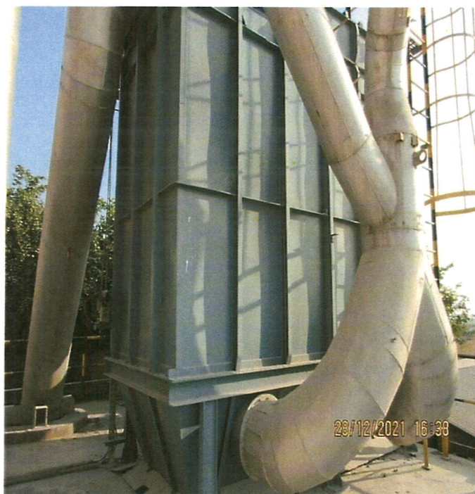
Image: Showing Dust extraction system to control fugitive emissions
